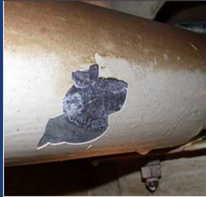
Film defect detachment
